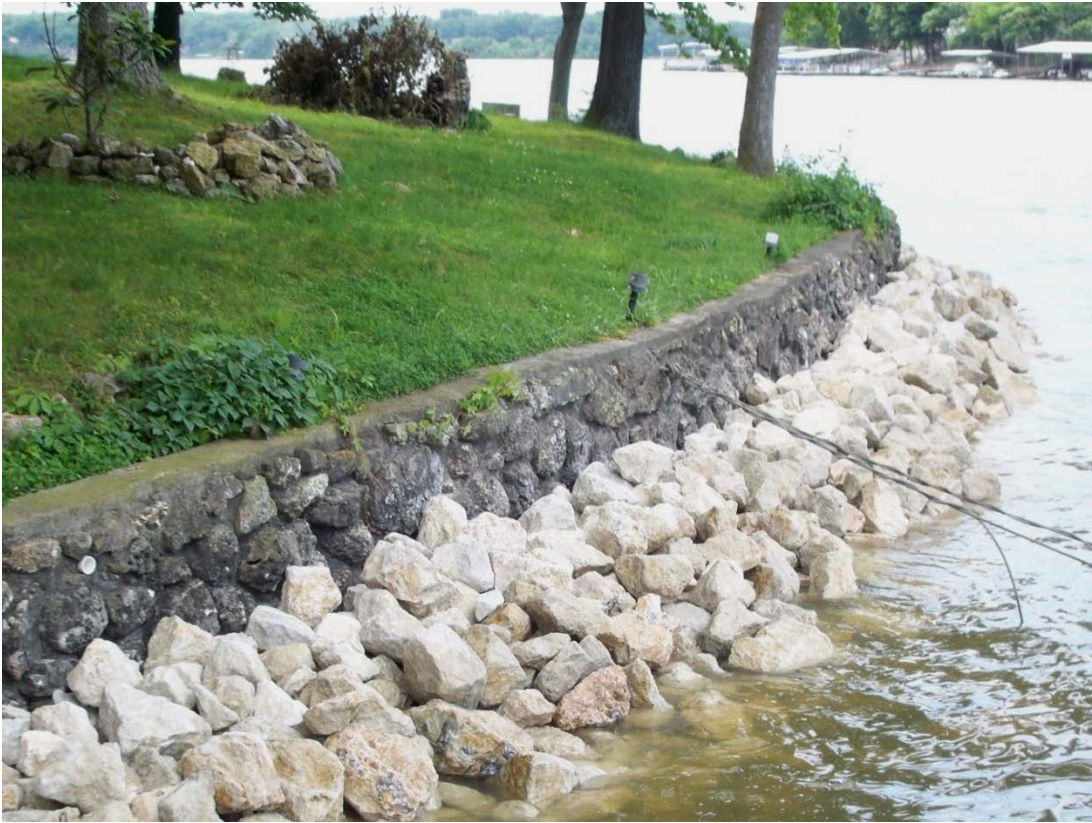
Figure VI-5a. Older seawall reinforced by riprap. Photo courtesy of Horseshoe Bend Dock and RipRap Company.
